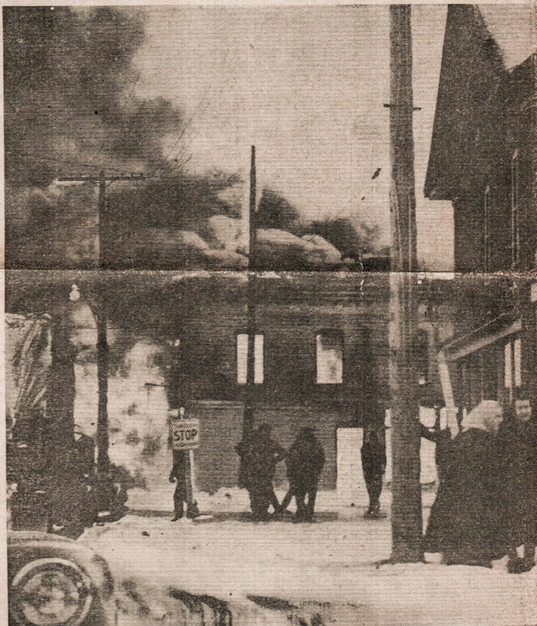
VILLAGE STORES, POST-OFFICE DESTROYED BY FIRE
