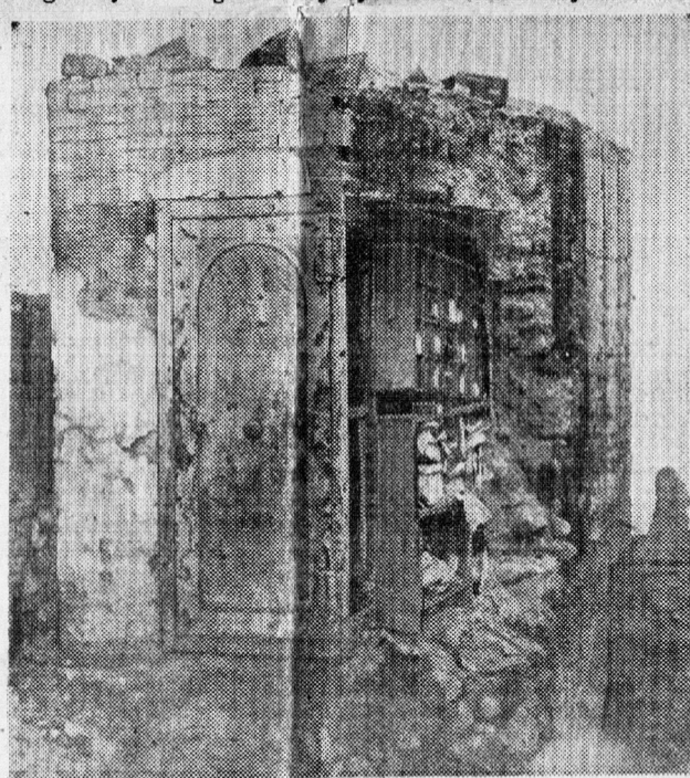
Post office fell before the flames but brick wall and sturdy door saved the mail, here shown in pigeon-holes ready for collection.
